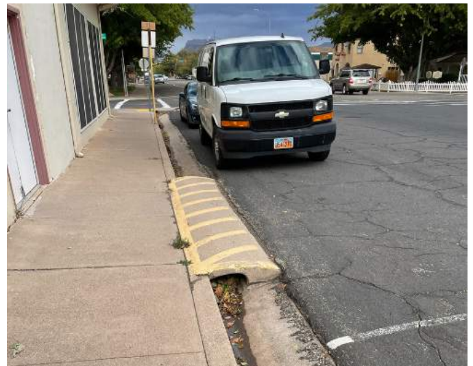
Sample access ramp in Hurricane
