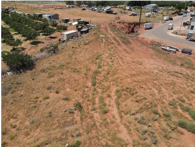
^Overhead view of the substation site taken from the North West corner facing South East.
