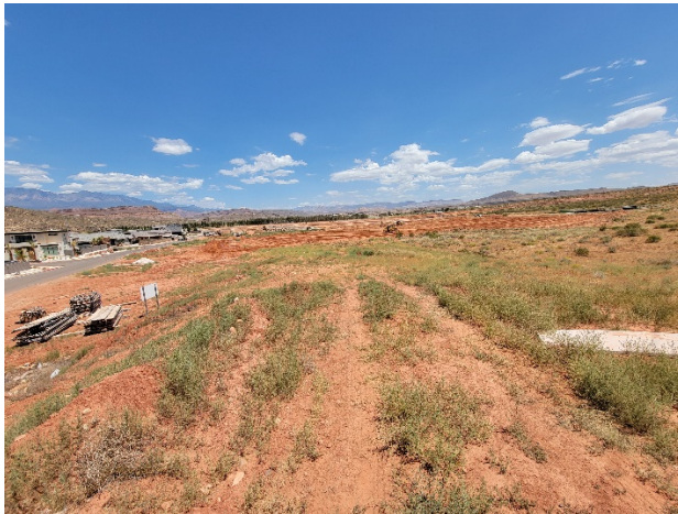
^South east corner of the substation site facing North.
