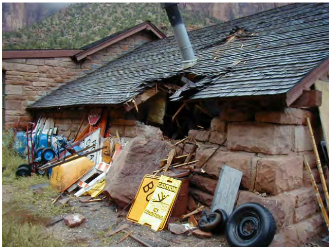
Figure 50. (A) Rockfall in 1947 through the roof of a maintenance building in Zion National Park. (B) Rockfall in 2010 through the roof of the same maintenance building. Photos courtesy of National Park Service.
