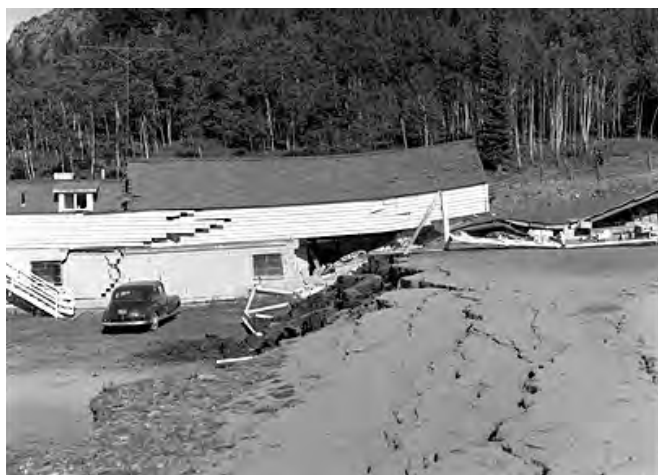
Figure 9. Normal fault surface-faulting damage to a building, 1959 Hebgen Lake, Montana, M 7.3 earthquake. (Photograph by I.J. Witkind, USGS.)
