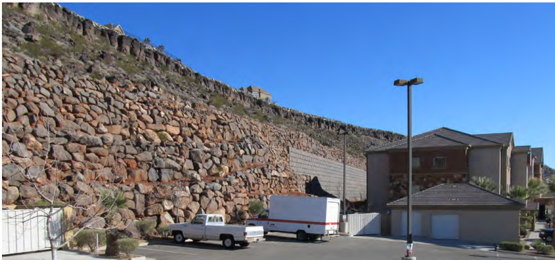
Figure 44. Unreinforced rockery wall typical of many constructed in recent years in Utah. Strong ground shaking during an earthquake may cause such walls to fail and generate urban rockfalls. Photo taken January 2013.
