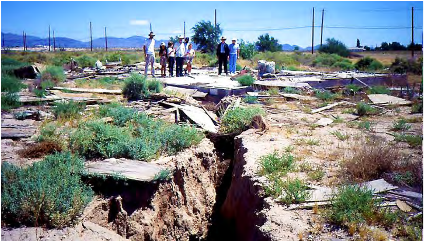
Figure 38. Remains of a home severely damaged by an earth fissure and eventually torn down in the Windsor Park subdivision, Las Vegas, Nevada.
