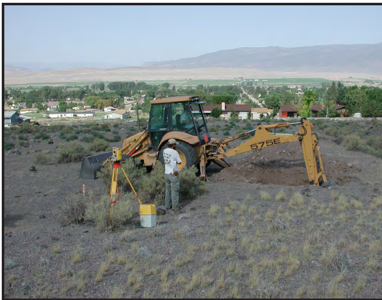
Excavation of a test pit for a geotechnical investigation in Utah.
