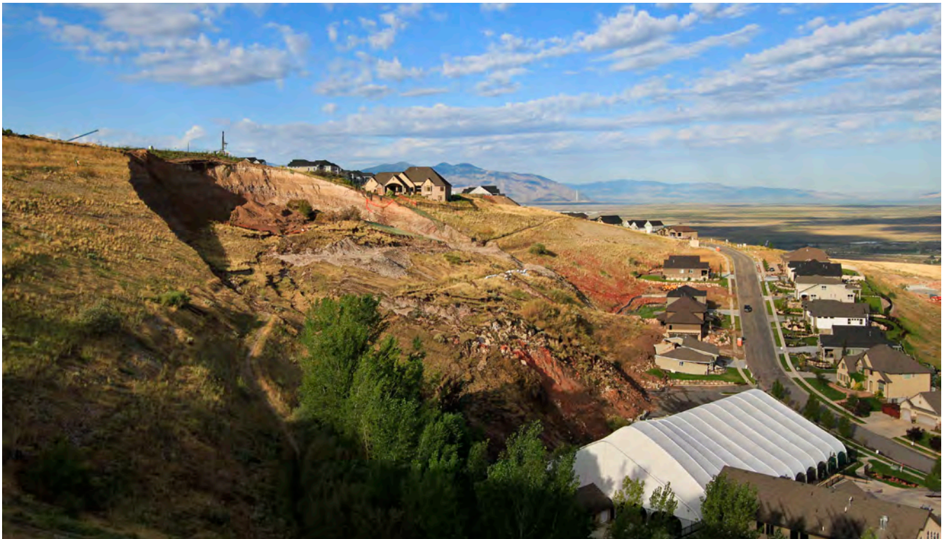
Figure 20. August 2014 Parkway Drive landslide, North Salt Lake, Utah. The effects of this landslide illustrate how damage can occur at various parts of the slide. The landslide severely damaged the Eagle Ridge Tennis and Swim Club (white tent structure), and one house (directly above the tent structure) at its toe, partially destroyed a home's backyard along its left flank (behind orange fencing near center of photograph), and threatened streets and pipelines near the crown. Photo date August 14, 2014.
