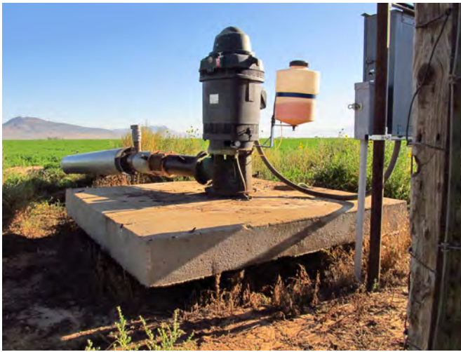
Figure 40. Protruding well head due to land subsidence resulting from groundwater mining. Photo taken September 2014.
