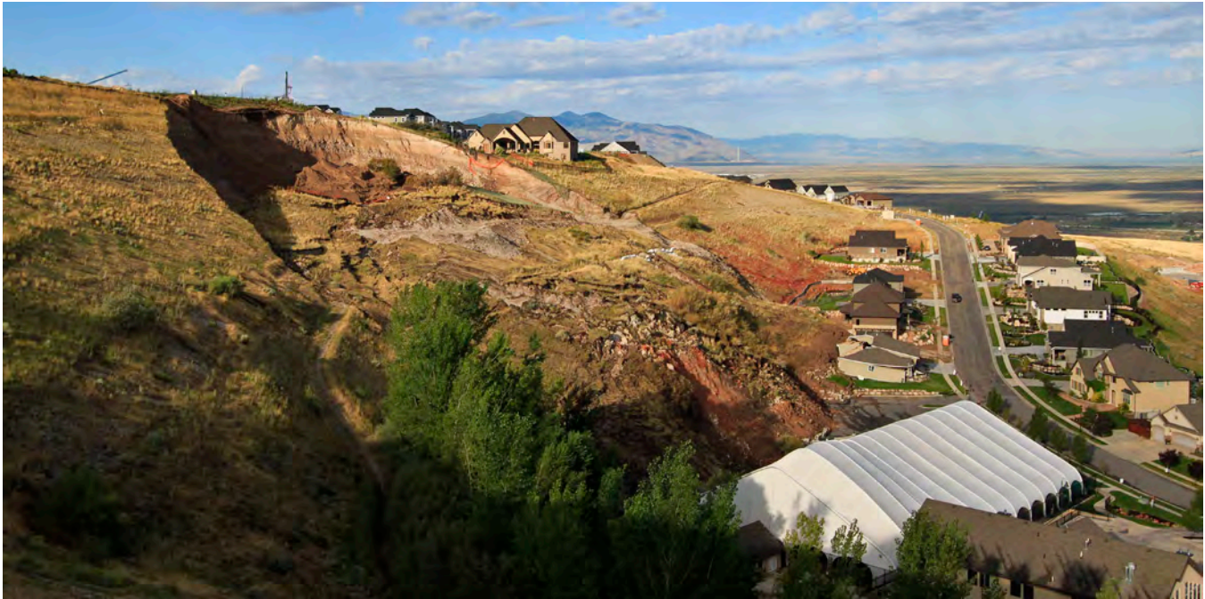
Figure 1. August 2014 Parkway Drive landslide, North Salt Lake. The landslide damaged the Eagle Ridge Tennis and Swim Club (white tent structure), severely damaged a house (directly above the tent structure), and removed part of the backyard of a second home. Photo credit: Gregg Beukelman, August, 14, 2014.
