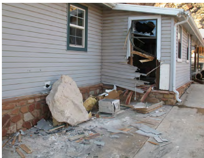
Figure 42. Rockfall damage to a house in southern Utah. Rockfall boulder leaning against wall passed entirely through the house and struck a vehicle in the driveway. Photo credit: Dave Black, Rosenberg Associates, photo taken February 2010.
