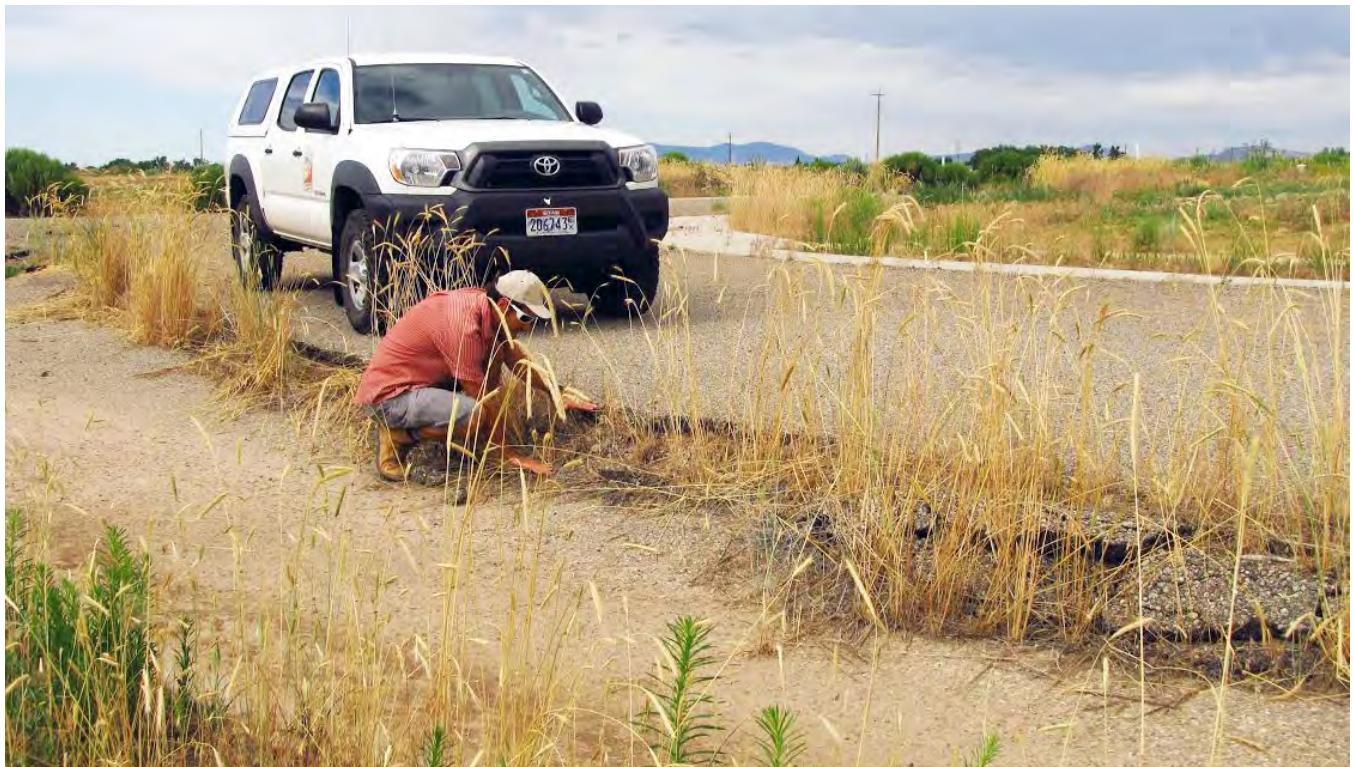
Figure 34. Damage to street pavement by an earth fissure in Cedar Valley across which differential displacement is occurring at a rate of about 2 inches per year. Photo taken July 2015.
