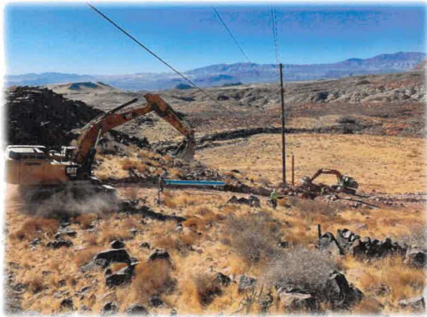
City Creek Pipeline Project; circa 2021
