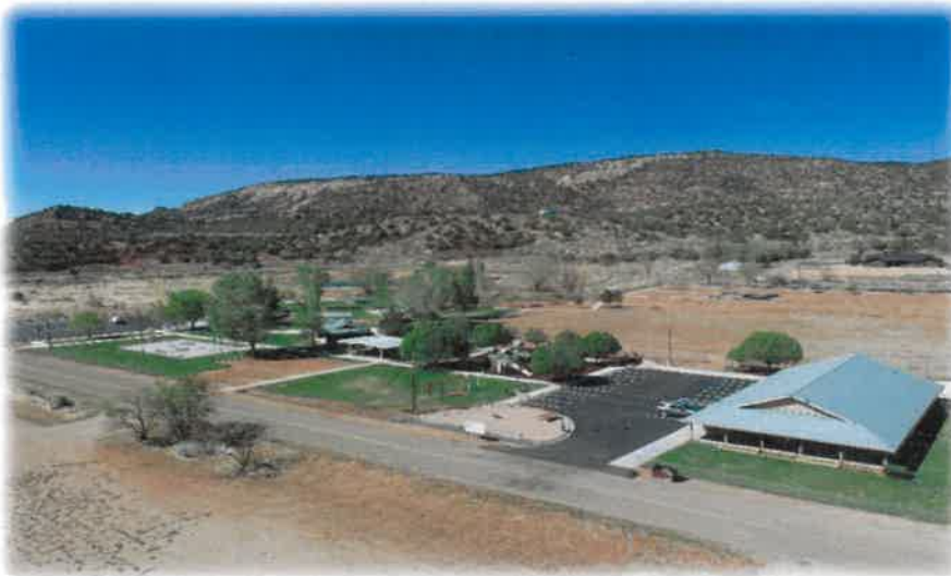
Kaibab Sidewalk-Paving & Park Improvements; 2021
