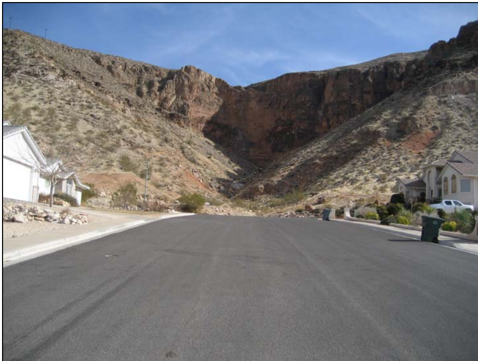
Figure 1-4 Hillside Development at 2050 South Street and Canyon Mouth With No Conveyance Facilities for Major Floods
