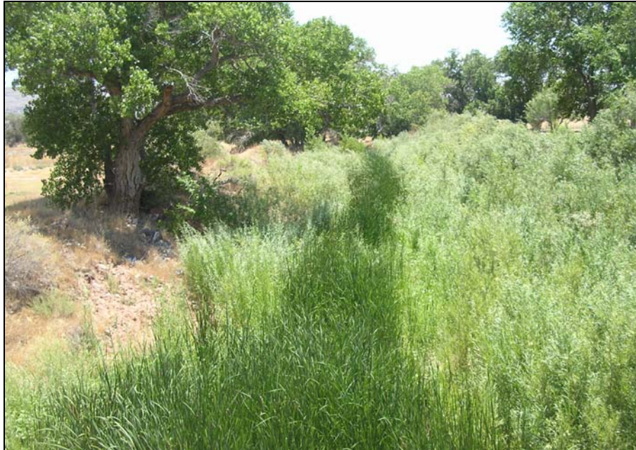
Figure 1-3 Vegetation growth in Gould Wash at State Street culvert looking upstream.
