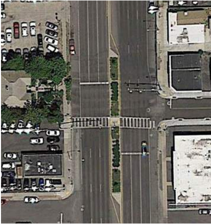
Aerial view of HAWK signal
