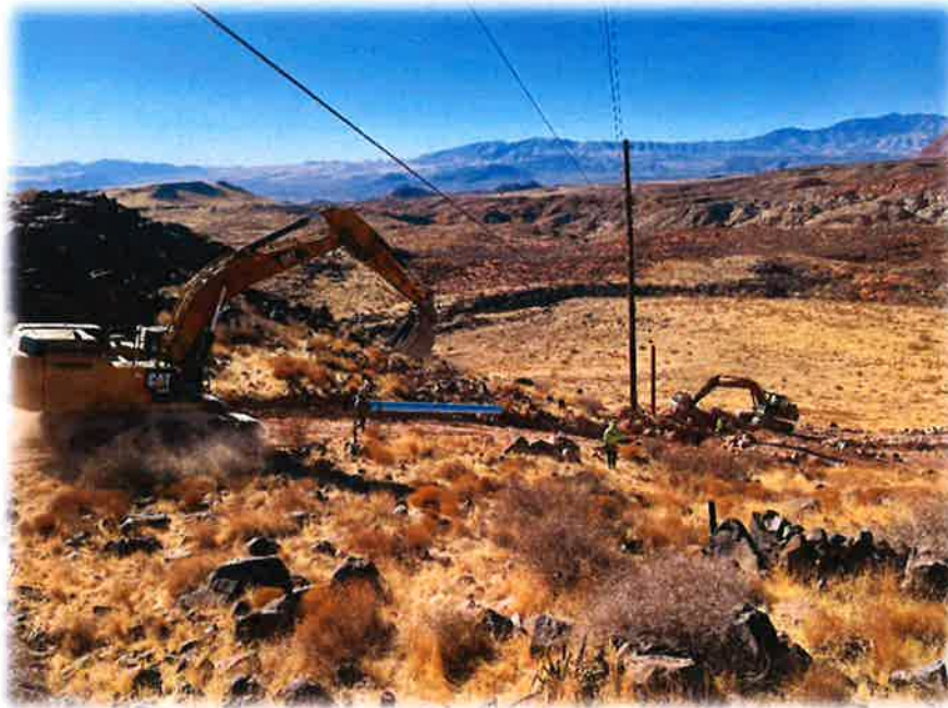
City Creek Pipeline Project; circa 2021
