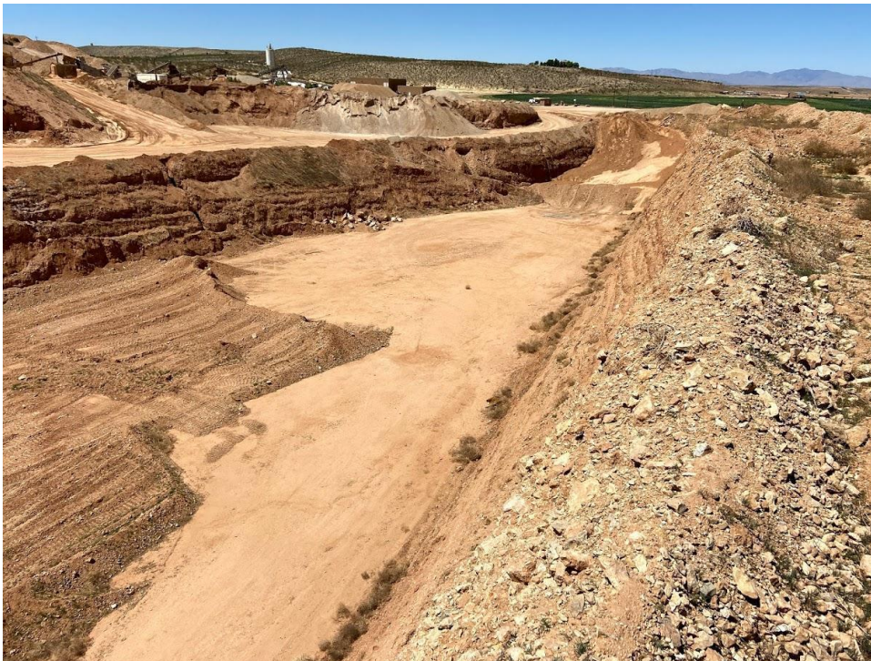
1100 W Gravel Pit Operation and Southern Border of this Zone Change Application
